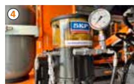
4 Central lubrication system
