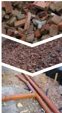
Refilling pipelines 0/64
