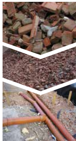
Refilling pipelines 0/64
