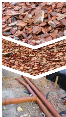
Refilling pipelines 0/64
