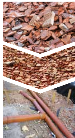
Refilling pipelines 0/64
